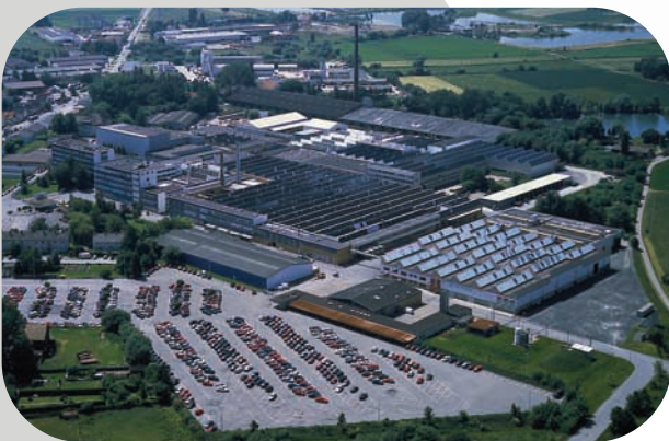
Stiebel Eltron's plant in Holzminden, Germany
